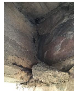
Spalling/scaling Exposing Rebar
